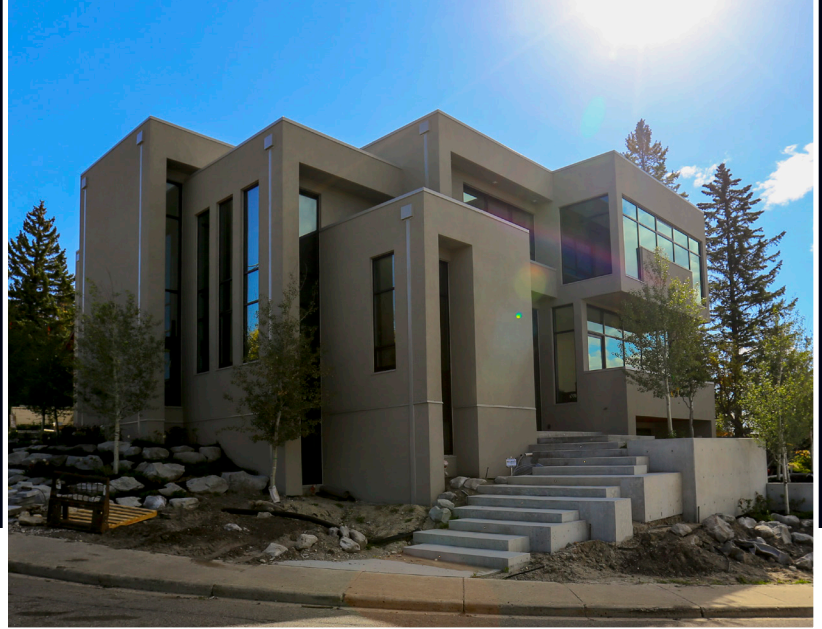
New construction with ShieldIt
