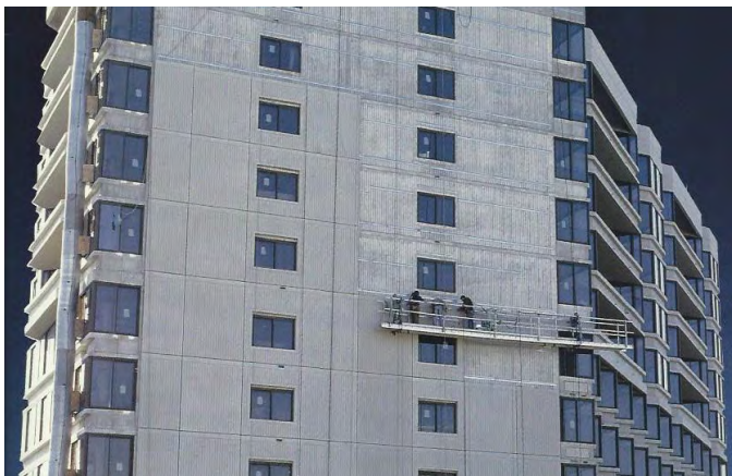
Fedderlite MP restoration over split-faced block
