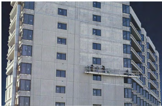
Fedderlite MP restoration over split-faced block
