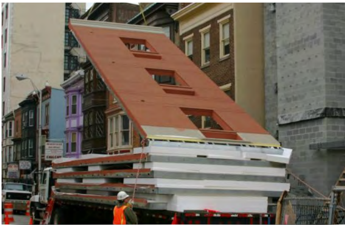
Outsulite panel installation
