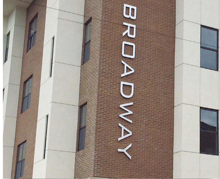
Office Building Schenectady, NY
